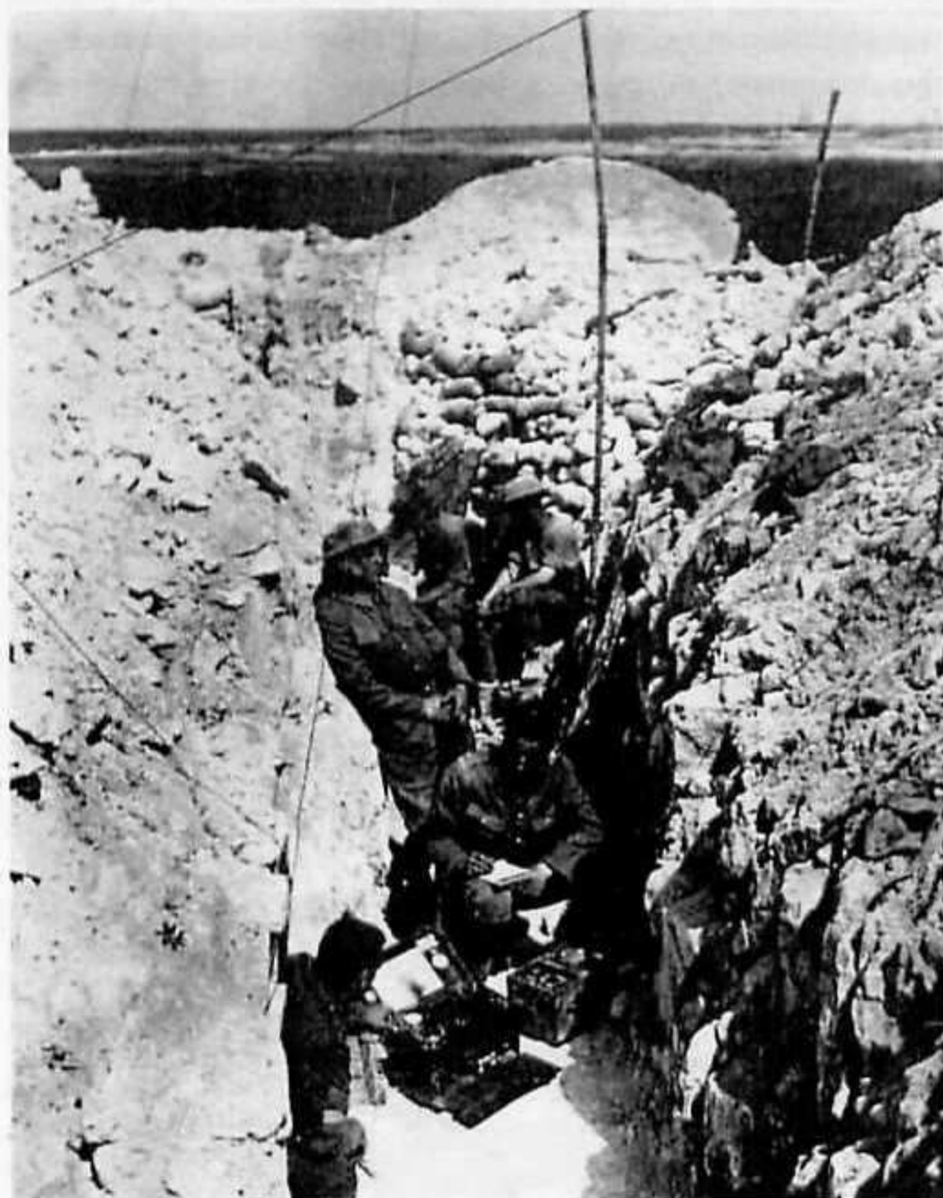
Fig.3. The BF Set, its aerial supports and 'Sparks' in a trench somewhere on the Western Front
